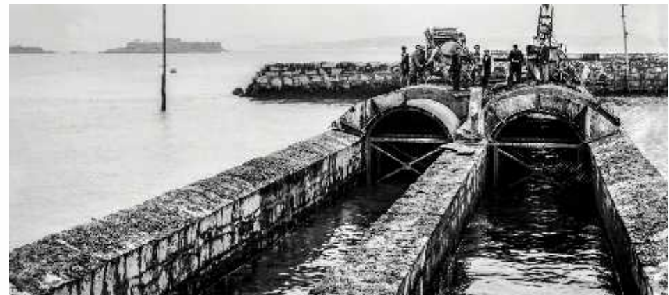
Construction of the sea outfall pipeline in 1931.
