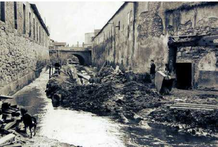
Channelling works. Oza Avenue Bridge (1966-1970)
