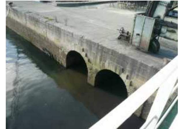
Current photograph of the outfall
